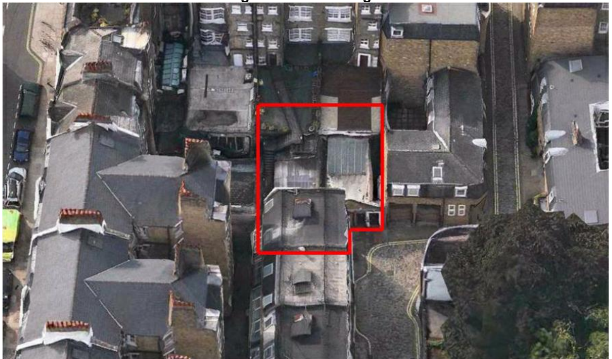
View south west: Charles Lane to right, Allitsen Road on the left
