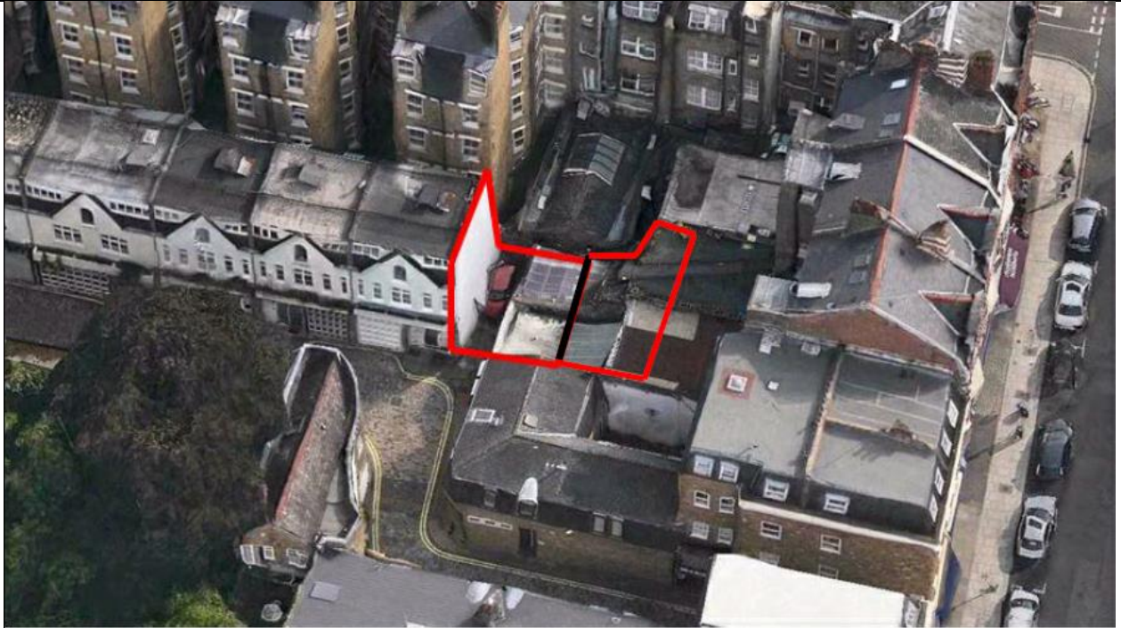
View south east: St Johns Wood High Street on the right
